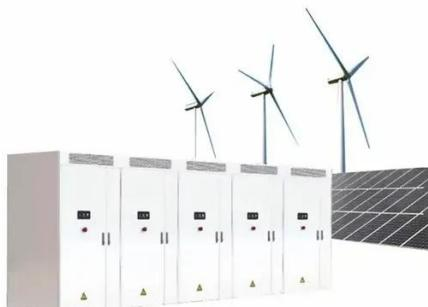
Inverters are the part of the solar array that connects to the step-up transformer. Inverters convert DC generated solar power into AC. ...
