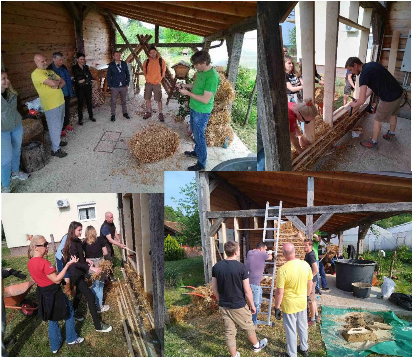
Pic.6. Participants of the workshop building the strawbale wall, "Hlinár" Stano Prorok
